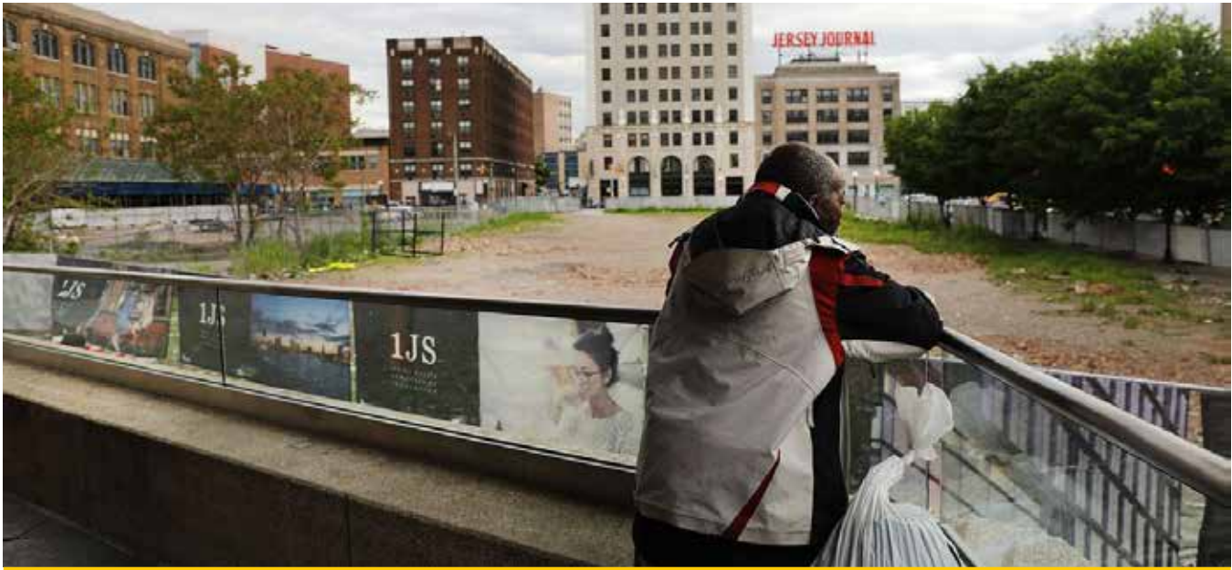
The site of Kushner Companies' One Journal Square luxury flat project in Jersey City in the northeastern US state of New Jersey. In 2017, the company marketed the project while promoting its connection to US President Donald Trump, leading to US prosecutors' investigation into the company and its tactics. Photo: AFP
